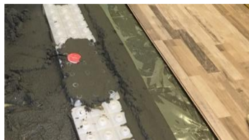
Figure 2: Floor installation, positioning of the heat flux meter
