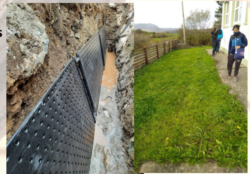
Left: Installation of the flat panel GSHX. Right: re-instatement of landscaping.
